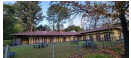
Cherry Hill Detox Facility Roof
