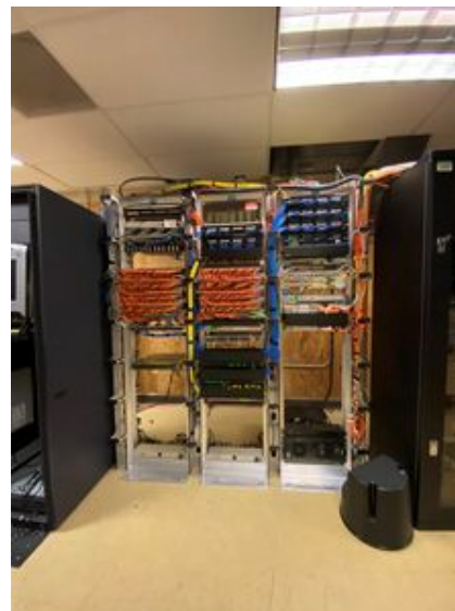
Gail Steele Multi Service Center Building Network Upgrades
