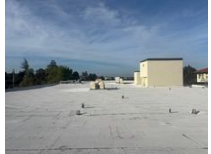
Fairmont Building H Roof
